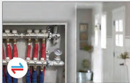
CEILING RADIANT SYSTEM
